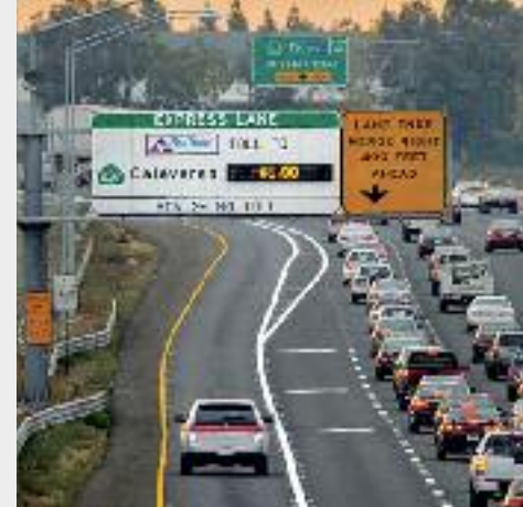
For paying customers, overhead electronic pricing signs will display current toll rates. (Photo: Noah Berger)
