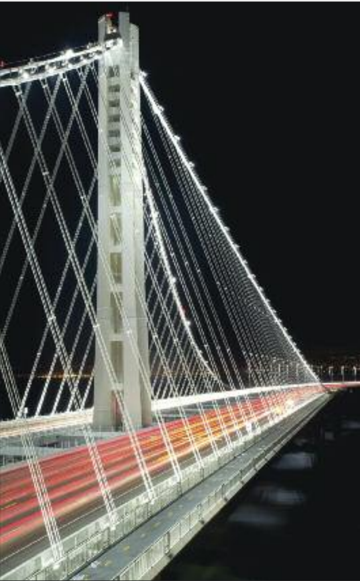
The New East Span of the San Francisco-Oakland Bay Bridge opened on Labor Day 2013. (Photo: Noah Berger)
