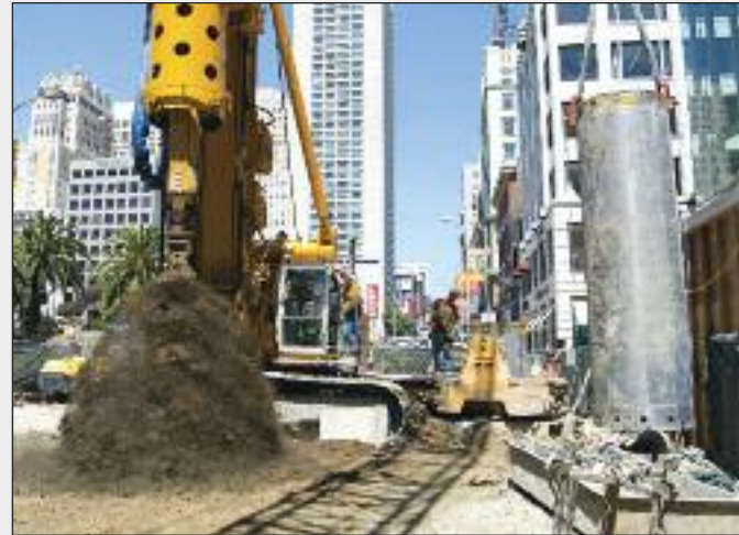
Construction underway in San Francisco's busy Union Square shopping district.
