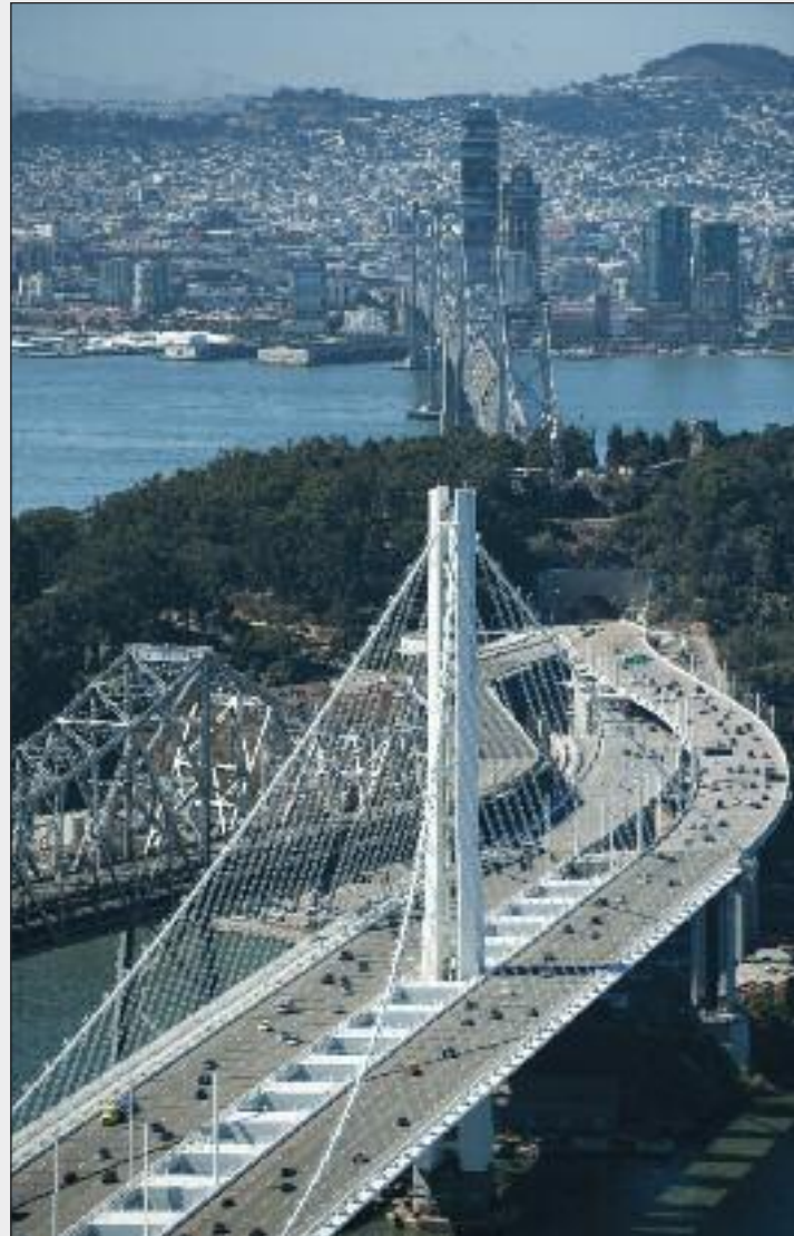
The TBSRP included both the new Bay Bridge East Span and a retrofit of the West Span. (Photo: ©Barrie Rokeach 2014, www.rokeachphoto.com )
