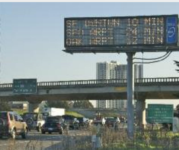
Changeable message signs help drivers gauge the amount of time a trip will take.
