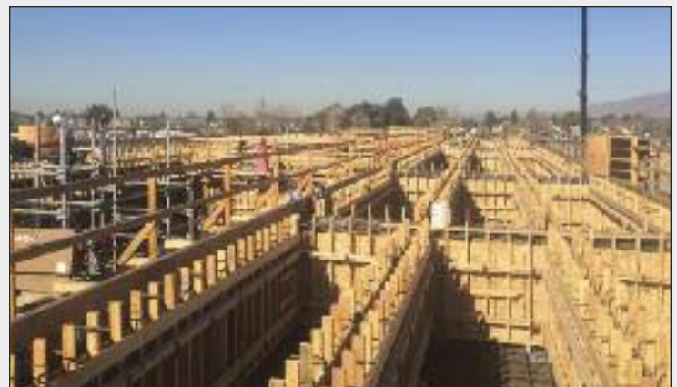
Formwork at the site of the Berryessa Station in San Jose. (Photo: Courtesy of VTA)
