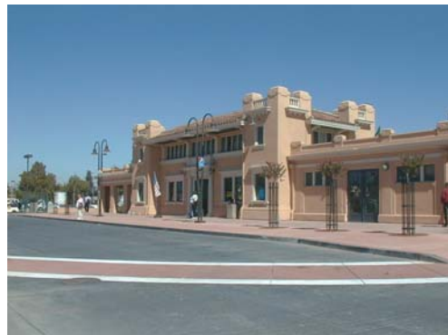
VTA's downtown Gilroy Caltrain Transit Center connects local bus and commuter train services.
