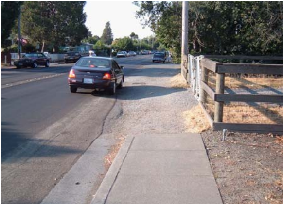
Discontinuous sidewalk network
