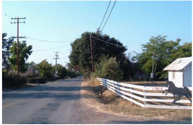
Lack of sidewalks on Burbank Avenue
