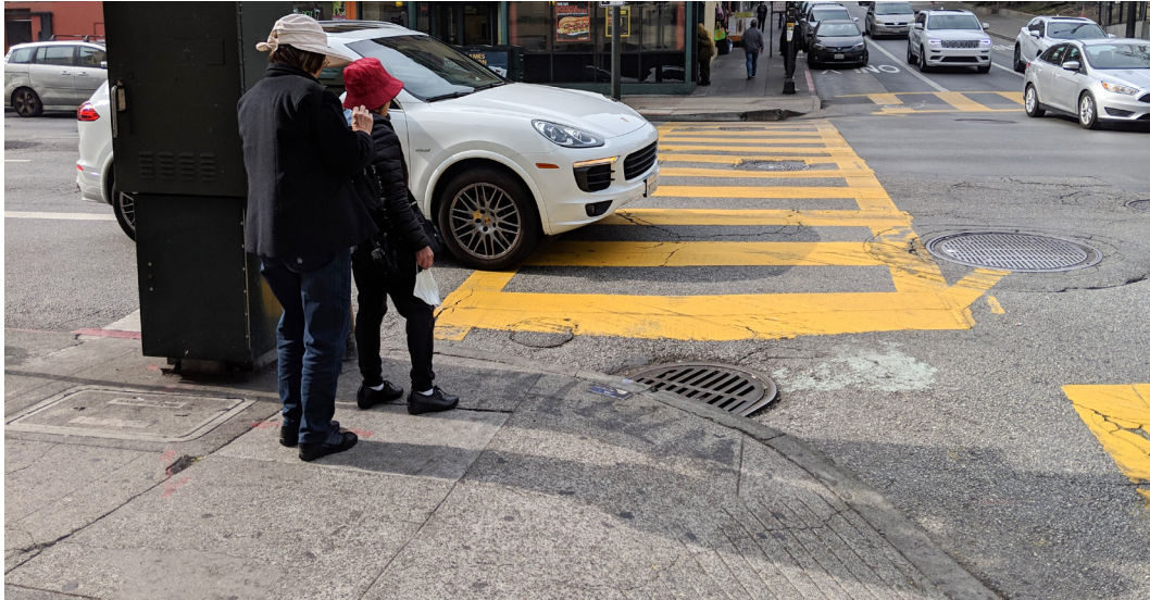
Figure 15. Missing Directional Curb Ramps at Kearny & Clay Due to Conflicting Inlets and Signal Equipment
