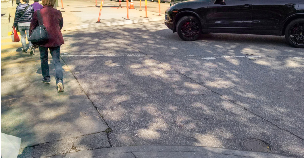
Figure 18. Dual Turn Lanes into the Portsmouth Square Garage Create a “Double-Threat” for Pedestrians
