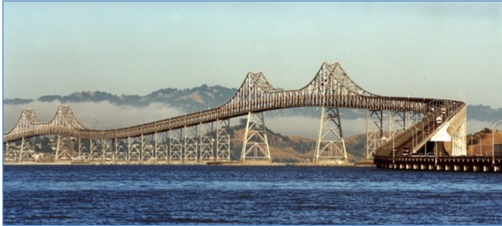
Figure 2-2: Richmond-San Rafael Bridge
