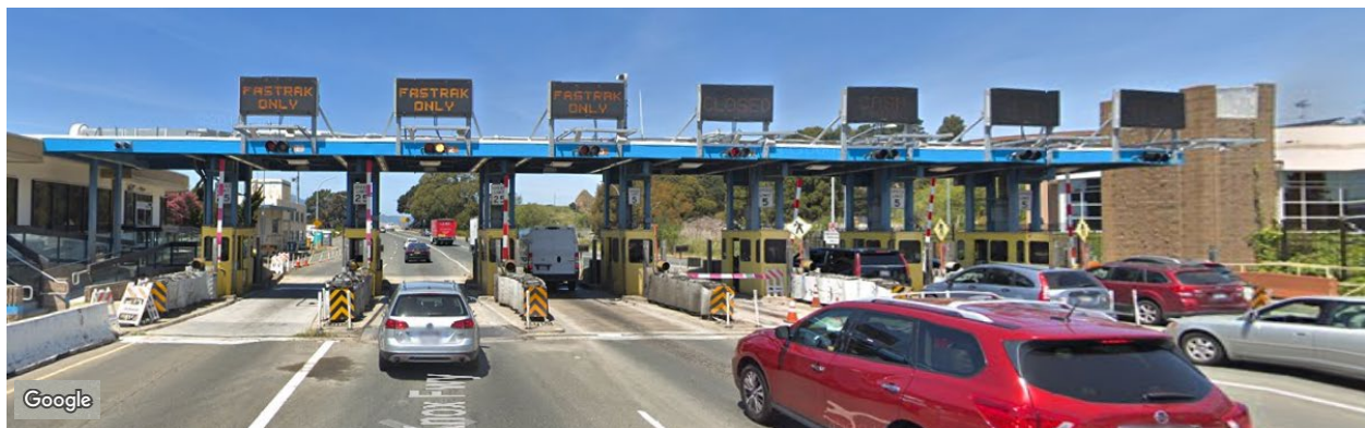
Figure 2-4: Approach to Richmond-Toll Plaza before March 2020
