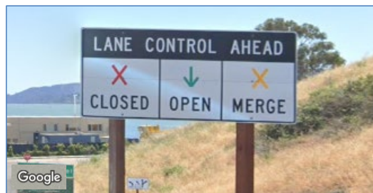
Figure 2-14: Sign Explaining Electronic Lane Control Displays
