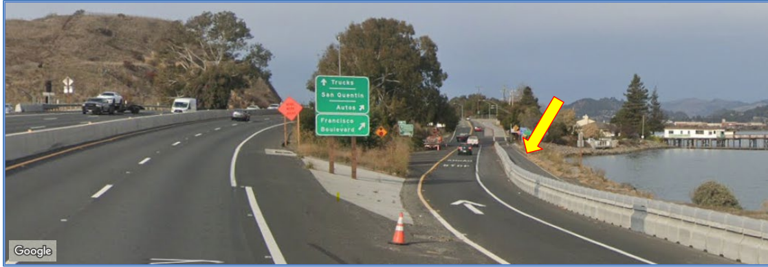
Figure 2-17: Bike Path Western End Along Main Street Off-Ramp
